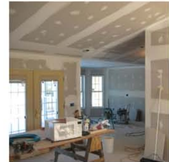
Drywall recently installed in a house.
